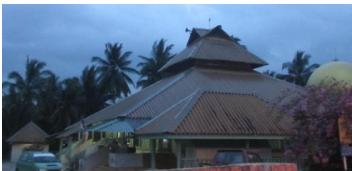
Figure 21: Three tiered roof Vernacular prototype/standard community Mosque of Pahang at Merapoh designed by Jimmy Lim Associates.
